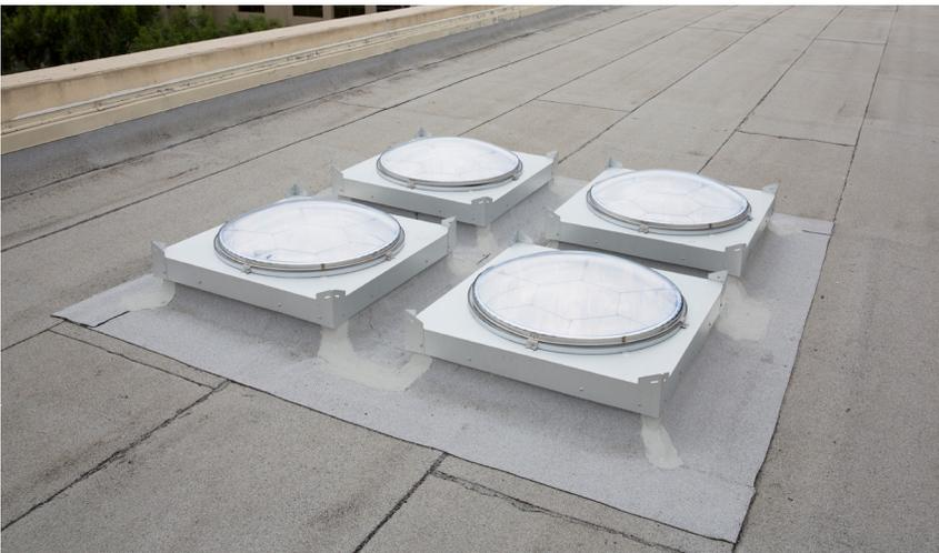
The unique installation included four (4) SkyVault M74 with Amplifier units, bundled together with a custom diffuser to provide maximum daylight. The installation was further customized with the installation of LEDs for both daylighting and night use.
