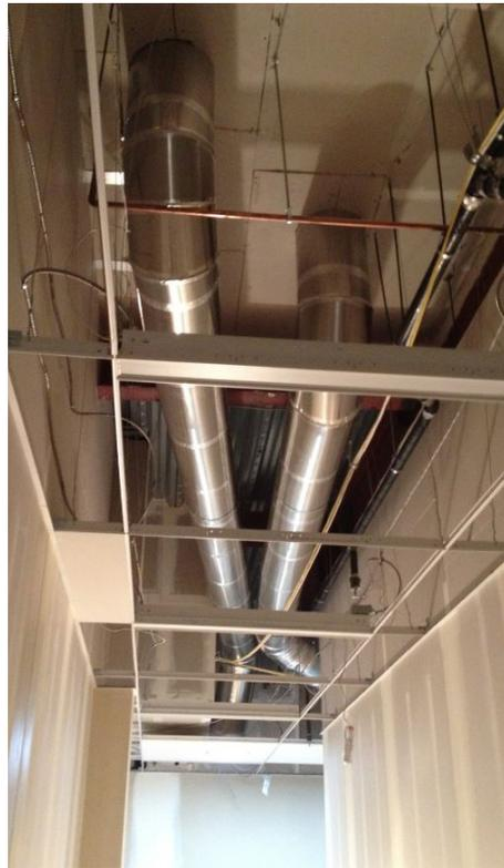
Typical commercial installations have tube runs of four to five feet. This project required horizontal tube runs of 17 feet, with minimal light loss.
